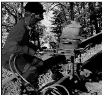
Thermit process for joining railway tracks
